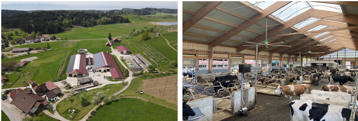
Figure 1: Study farm in the Lake Constance district in Baden-Württemberg, Germany with newly built dairy cow barn with membrane light ridge in comb barn (© B. Benz)
