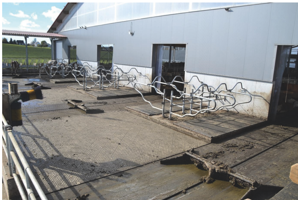
Figure 2: Structured exercise yard of the test farm with manure removal axles and turning flap turn scrapers
