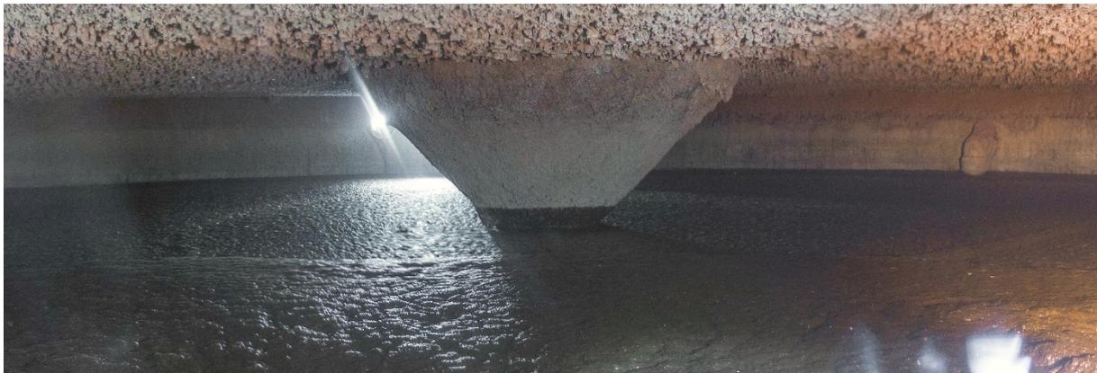
Figure 1: Inside view of the fermenter. Through microbial degradation of the hydrogen sulphide, deposits of elementary sulfur are deposited on the ceiling. © State Institute of Agricultural Engineering and Bioenergy, University of Hohenheim.
