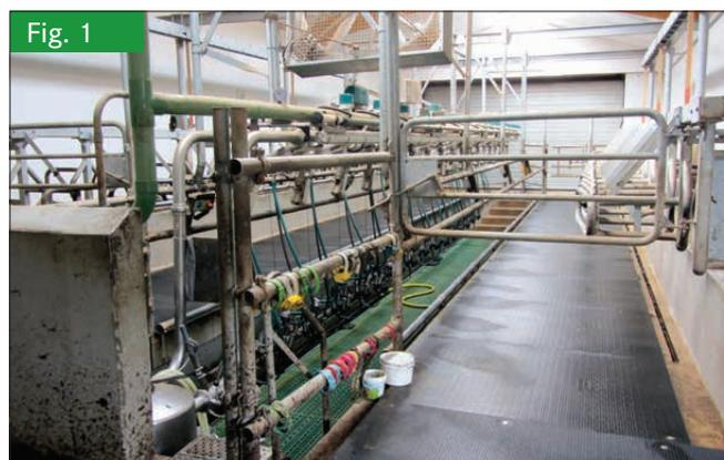
Fig. 1: Elastic flooring in the herringbone parlour with fast exit (Photo: B. Benz)
