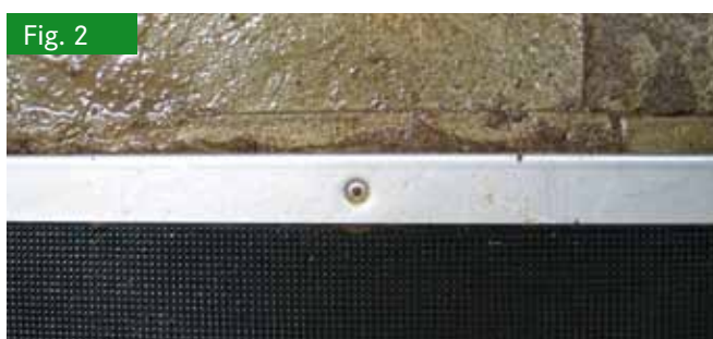
Fig. 2 Fastening of the stainless steel bar
