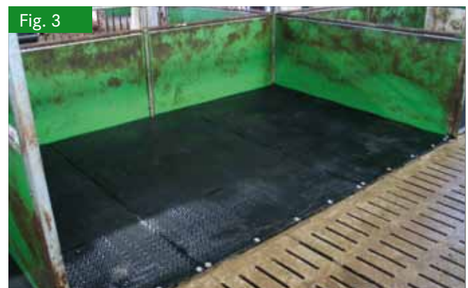
Fig. 3 Rubber mat with profile „hammer blow” and hard rubber edge
