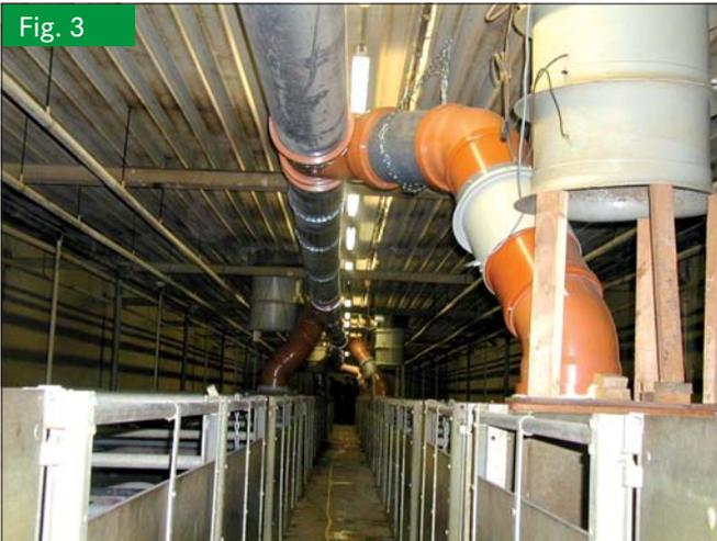
Study design with simultaneous above- and under-floor suction. Air is withdrawn both beneath and above the floor (at a set distance from the ceiling)
