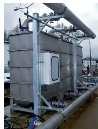
Desulfurization system of a biogas plant (2 MW<sub>el</sub>) (source AdFiS systems GmbH)
