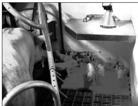
Fig. 2: Warm water underfloor heating combined with infrared lamp in the piglet creep lid
