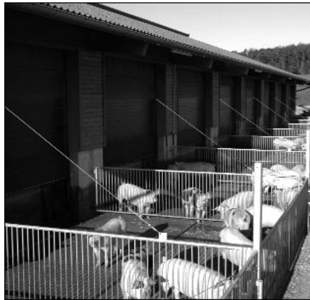
Fig. 3: Feeding pig housing with natural ventilation
