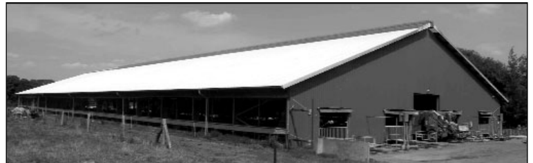
Fig. 1: Exterior view of the cow barn from the south
