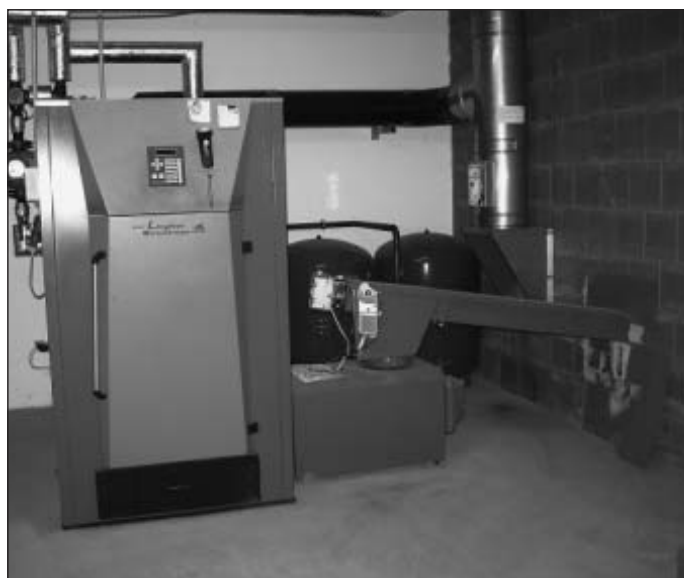
Fig. 2: Wood chips furnace: automatic furnaces for wood chips are almost technically mature.
