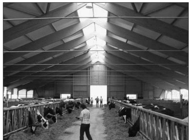
Fig. 1: The self-supporting construction with inconspicuous tensile beams gives a light and airy impression in this barn owned by the Dörr family.
