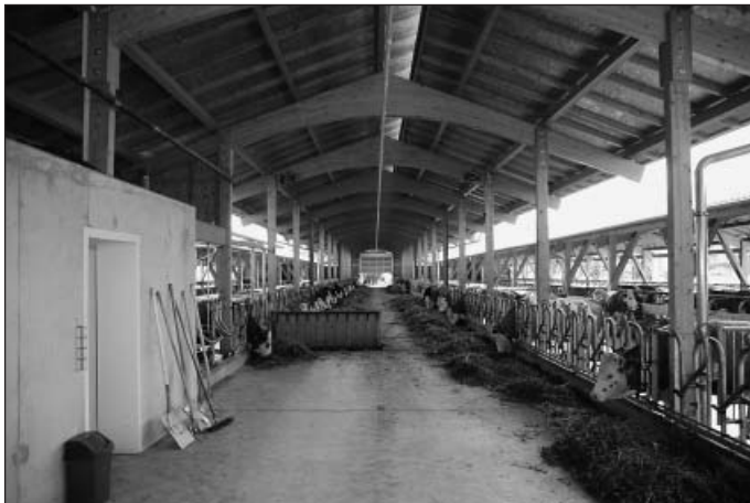
Fig. 2: The Kűfner and Naiser partnership planned its cubicle house as a three-barn complex whereby timber cross sections worked out relatively small.
