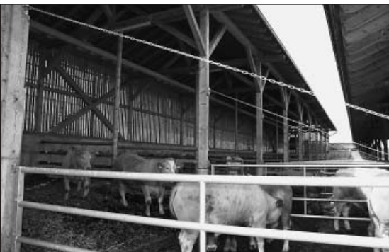
Fig. 5: For beef cattle the Schmid family built straw yards and for dairy cows cubicle housing on both sides of a roofed feeding passage.
