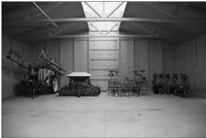
Fig. 4: Three-ply panels with laminated timber frame ribbing are basic elements brought together in the construction of Johann Kinzner's machinery barn.
