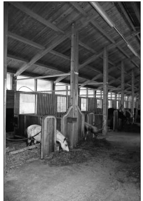
Fig. 6: Special front walls with feeding slits and removable horsebox side walls bring considerable labour savings in the stable built by the Staud family.
