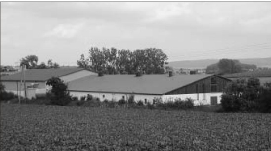
Fig. 1: With larger livestock housing the trend is towards decentralised exhaust air solutions.
