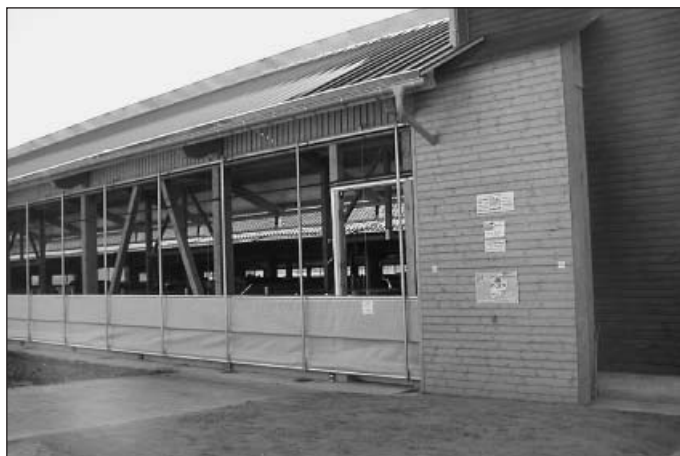
Fig 3: In many cases mechanically adjustable side screens have become established for aeration control in naturally ventilated barns.
