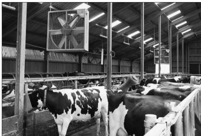
Fig. 4: Fans built into naturally ventilated barns reduce heat stress in summer.
