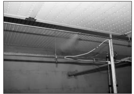
Fig. 2: Fogging can sink barn interior temperatures by up to 5°C.
