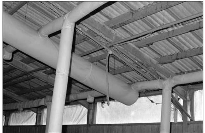
Fig. 2: Sectional view of the system for tracer gas injection with main-distributor, by-distributor and two vertical outlets
