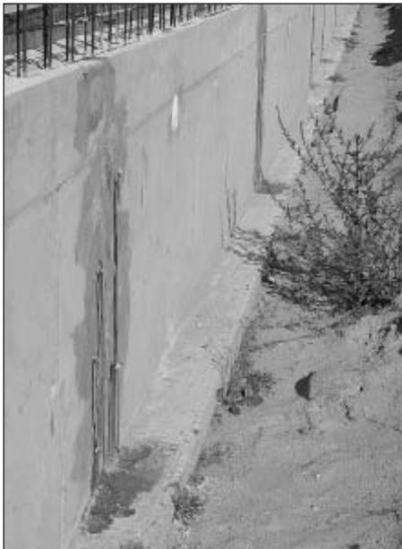
Fig. 1: Leakage in a newly built slurry channel
