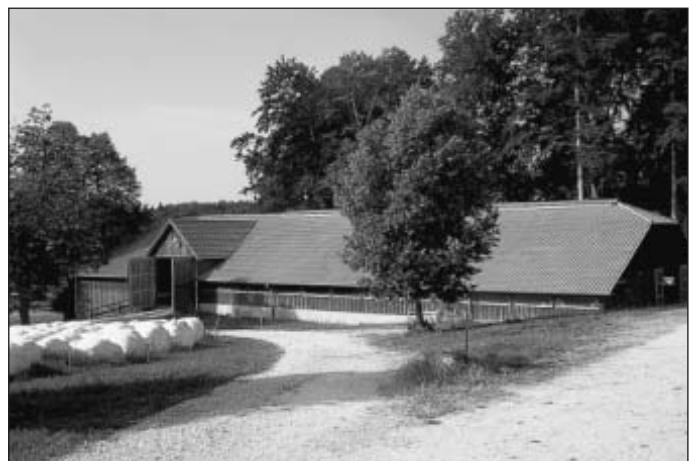
Fig. 1: Sheep stable typical for the countryside with half-hip roof and standing dormers
