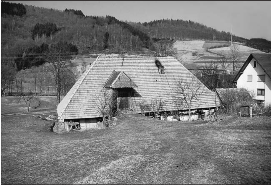
Fig. 2: The Black Forest farm building however, located at a slope, was accessed from the adjoining hill areas for storage goods. The regionally bigger snow masses, which covered the building in winter metres high, required an additional access from the lower side, which temporarily was only possible through a necessary balcony.
