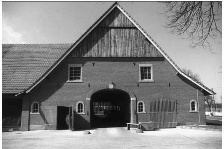
Fig. 1: In Lower Saxony you access the building through a big door at the ground level into the hall-way. Straw and other material for storage were transported up to the hall-way ceiling and simultaneously contributed there to heat insulation for men and animals living below.
