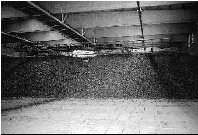
Fig. 2: Bulk store under roof with under floor ducts for ventilation
