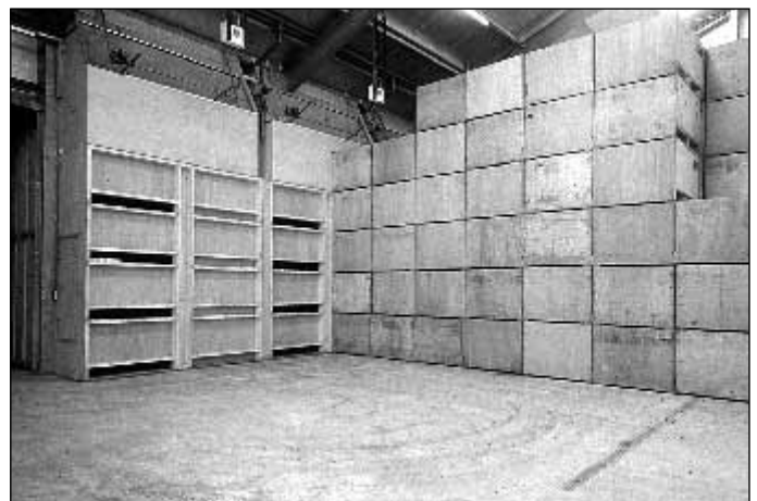
Fig. 3: A pallet box store with forced ventilation system
