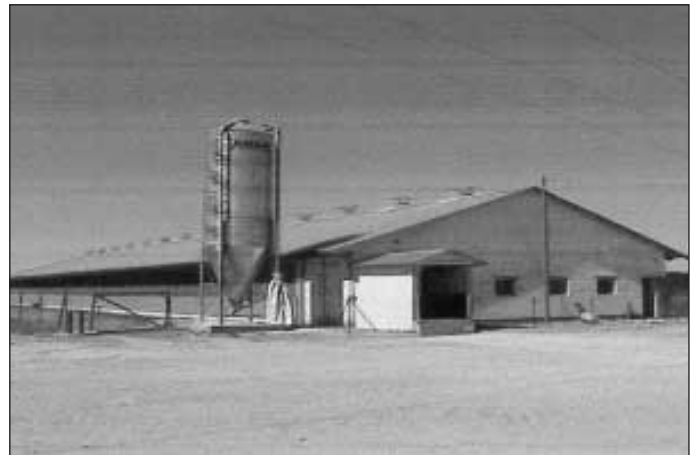
Fig. 3: Open stable with long sidewall openings (Nürtinger System)
