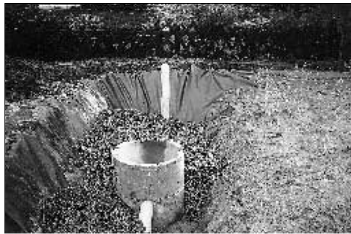
Fig. 2: Building wastewater plants with own-labour must be carried out very carefully
