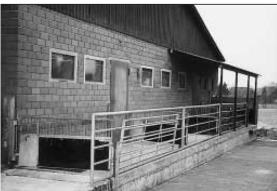
Fig. 1: Covered ramp with option for dividing and draining away from the house
